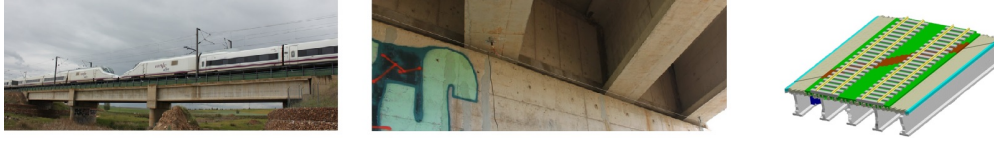
Figure 1: From left to right: Lateral view of the bridge. Diaphragms details. Numerical model.
